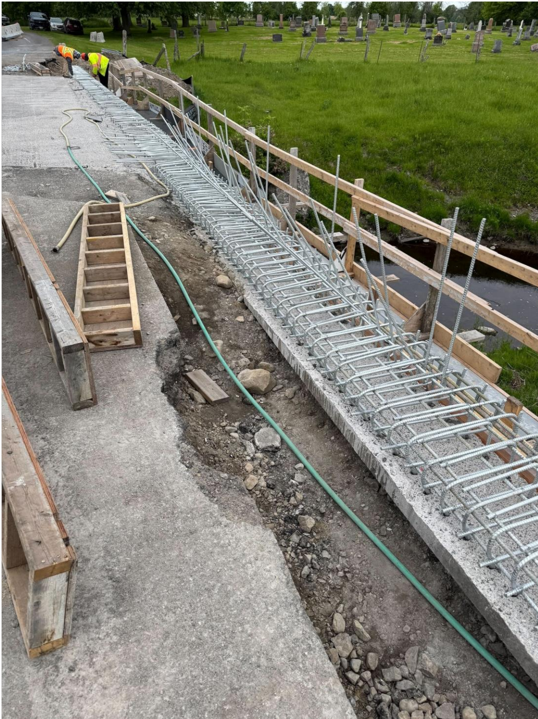
New Galvanized Steel Installation
