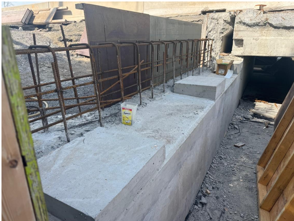
Newly Reconstructed Abutment Top and Bearing Pedestals
