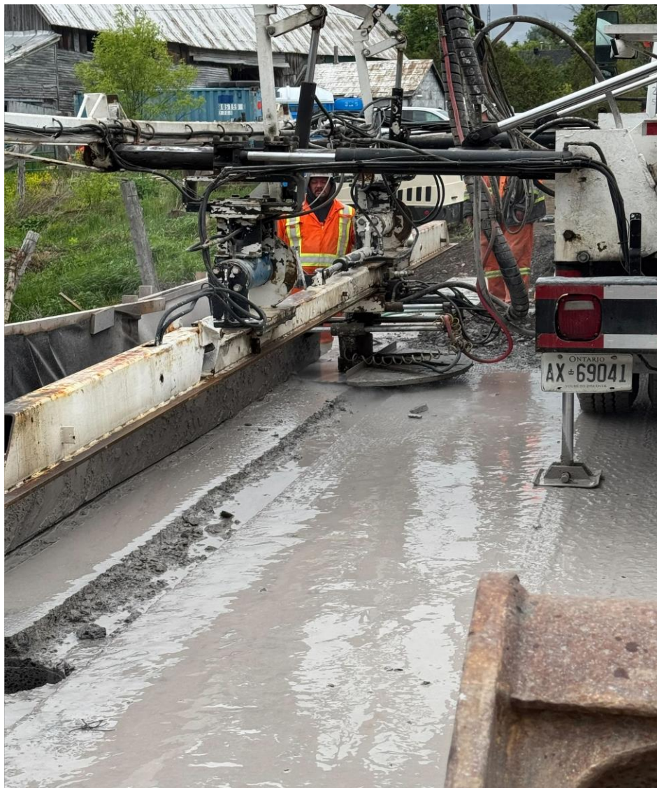
Stage 1 – Saw Cutting Removals
