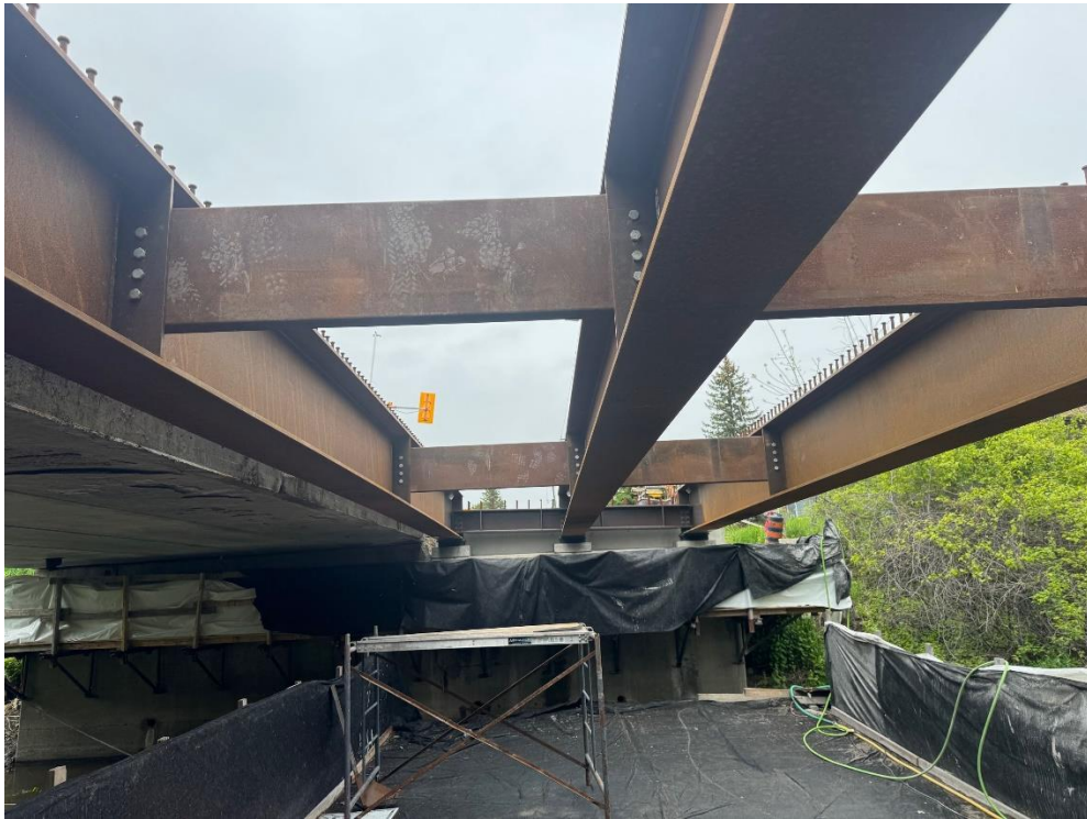
Newly Installed Stage 1 Plate Girders and Diaphragms
