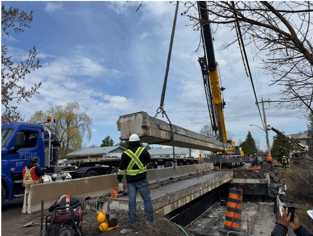
Stage 1 Girder Removal
